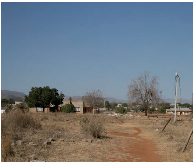
Disconnected electricity supply in Ga-Pila
